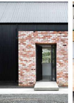
laps. Bricks from a warehouse that was a of the Christchurch earthquakes and had found their way to a local demolition yard were picked up cheap and seemed a fitting cladding of the block forms to the south side. They create beauty and contrast against the form of the steel cladding. A secondary barn clad in Dimondclad Rib 50 forms the garage, which is detached from the main building.
