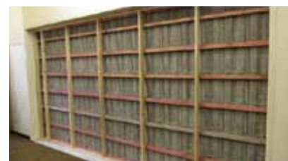
Concrete tiles from inside
