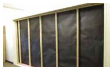
Underlay installed
