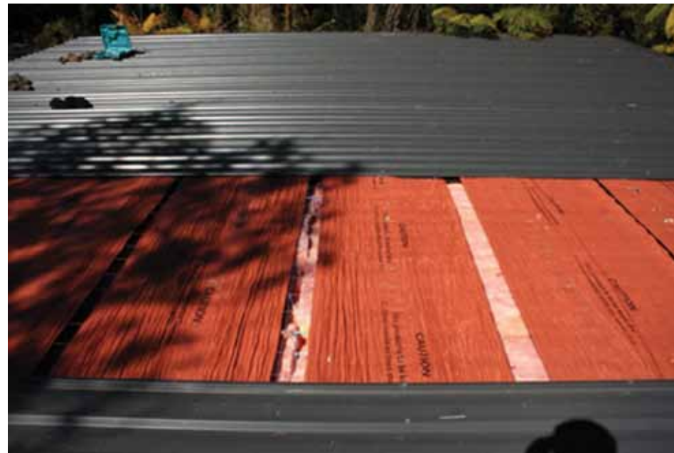
This 'concertina' result happened because the underlay was not 'captured at each edge by the fasteners at the purlins. That is why the 1200mm spacing must be reduced by the lap (150mm) = 1100mm for a 1250mm wide underlay.
