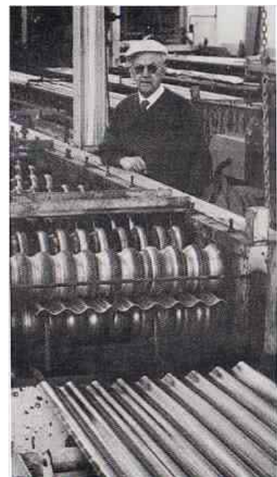
Auckland's rollforming pioneer, Nes Irwin beside the machine he built to produce New Zealand's first long-run corrugated iron. Photo © J.E.Farrelly
