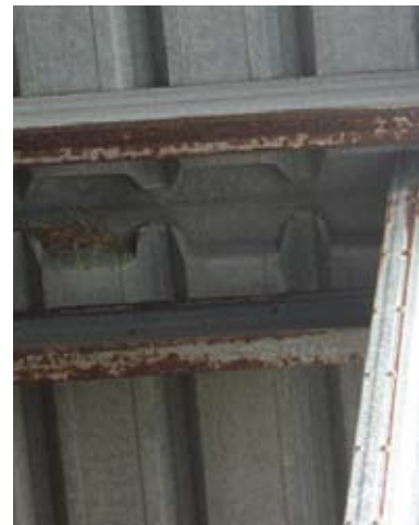
build-up of pre-treatment, primer and top coat at the extreme edge of the sheet.
