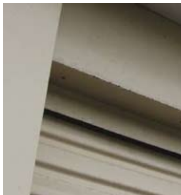
build-up of pre-treatment, primer and top coat at the extreme edge of the sheet.
