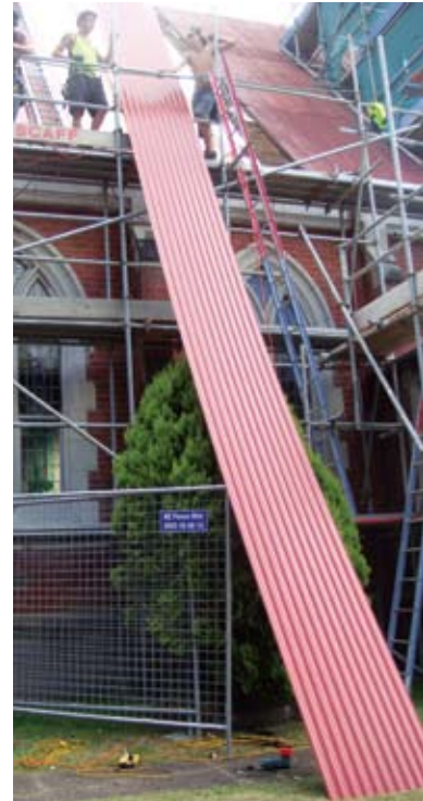
These Colorcote® ZRX Corrugate sheets were manufactured to size by Roofing Industries, Auckland, reducing waste. The 50 year old metal roof was removed and recycled.
