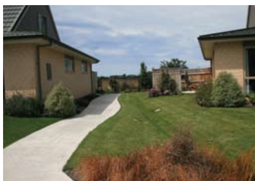
The grassed area (centre) is the only visible sign of the swale filter system that prevents sediment from entering the wetlands
