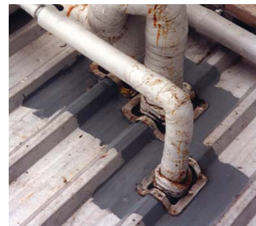
Where plant room supports are required to penetrate the roof cladding the designer should provide support framing from CHS.
