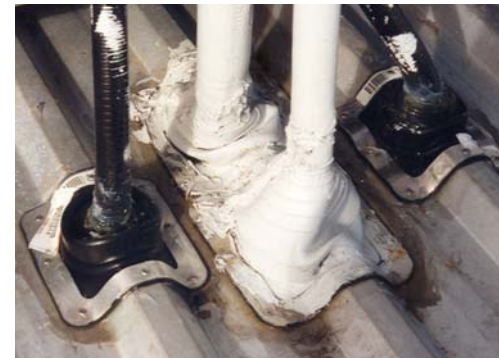
A Diverter or Cricket flashing designed to avoid build up of debris behind the back of a square or rectangular penetration.
